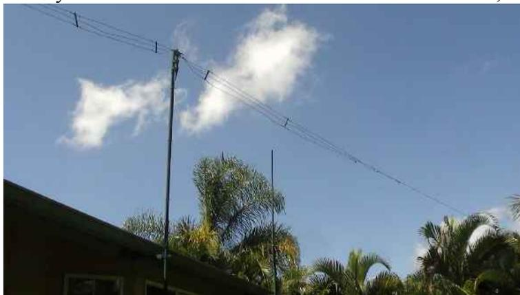
Fig. 15 15ft. mast on left is the center support for the Alpha-Delta DX-EE antenna. Vertical antenna and mast on the right is 2m/70cm Diamond X-50NA antenna.
