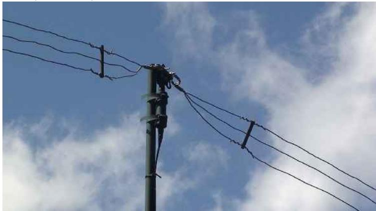
Fig.14 Close up detail of the center feed point for the Alpha-Delta DX-EE antenna. Immediately below the center insulator is an Unadilla W2AU, 1:1 BALUN.
